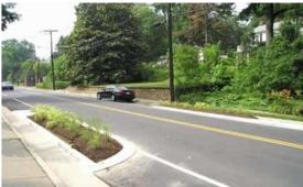
(g) <u>Chicanes</u>:- Chicanes is a series of attending mid-block curb extension or islands that narrow the roadway and require vehicles to follow a curving S-Shaped path, in the process the driver has to reduce the speed of his vehicles.
