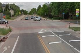
(f) <u>Chokers:</u> Chokers are Curb extensions that narrow a street by widening the side-walk on planting strips, affectivity creating a pinch point along the street. Choker can have a dramatic effect by reducing a two-lane street to one lane at Choke point.
