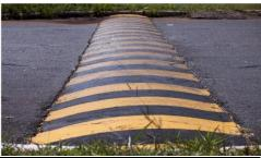
(b) Rubber/ Rumble Strips: - It is a corrugated pavement that causes rumbling sound and vibrations when vehicle passes over it; this alerts the driver to caution him to reduce his speed him to. It can be used on all Highways.
