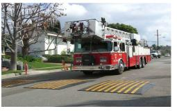
(d) <u>Speed tables</u>:- Speed tables are midblock traffic calming devices that raise the entire wheel base of a vehicle to reduce its traffic speed. Speed Tables are longer then speed humps and are flat-topped, with a height of 3-3.5 inches and a length of 22 feet. Vehicle operating speeds for streets with speed tables range from 40 KPH, depending on the spacing.
