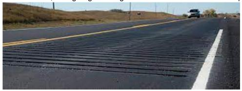
(j) <u>Optical Speed Bars</u>: Optical Speed Bars are transverse stripes spaced at gradually decreasing distances. The rationale for using them is to increase driver's perception of speed and cause them to reduce their speed.
